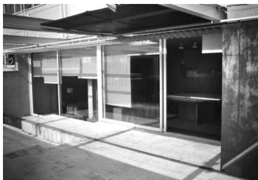
Figure 4 Porch of Corrales House. Filter and steps.
