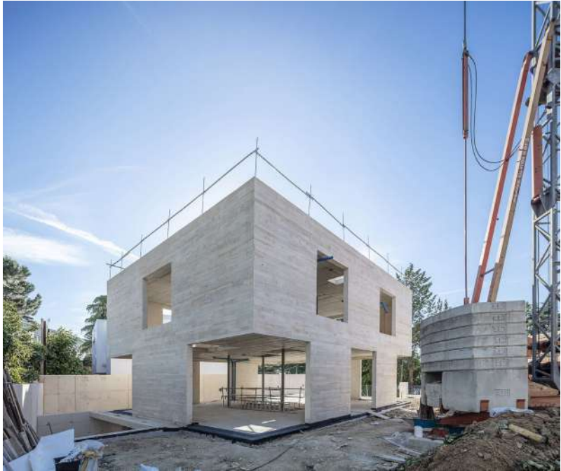
Figure 3 Domus Damero, 2019-2021, under construction, Jesús Donaire. Photography by Montse Zamorano
